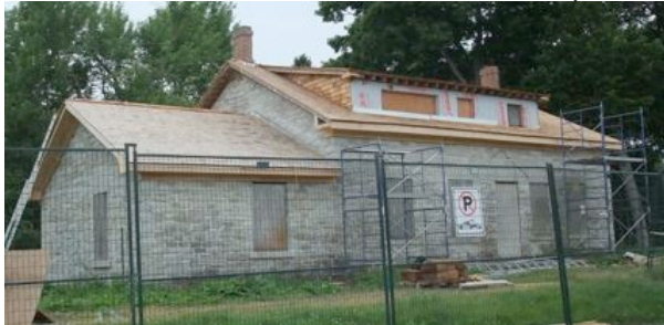
Wartman House with its new roof and woodwork/ Helen Finley 2011
