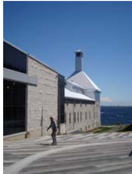
West Façade of the Tett Centre for Creativity & Learning / Paul Christianson, 2015
