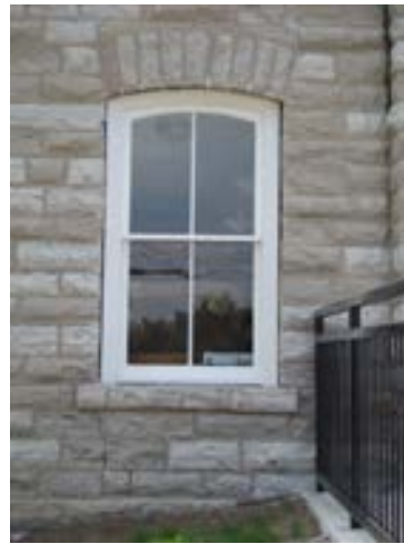
Detail of Window on Entrance Façade / Paul Christianson, 2015
