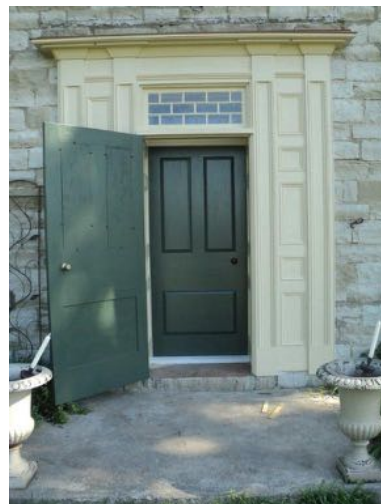
4106 Boyce Road—storm door and front door/ Photograph courtesy of Ron Tasker
