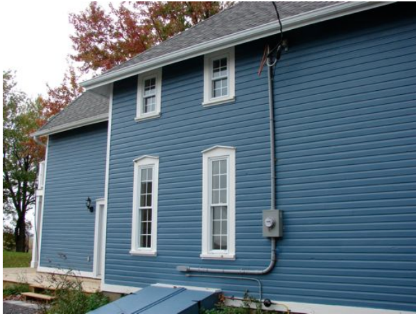
Restored Window Trim, East Façade, Nielson House/ Paul Christianson 2010
