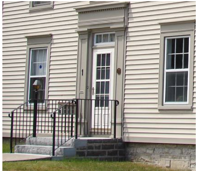
1 Baiden Street—detail of steps/ Paul Christianson 2016
