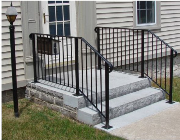
1 Baiden Street—detail of steps/ Paul Christianson 2016
