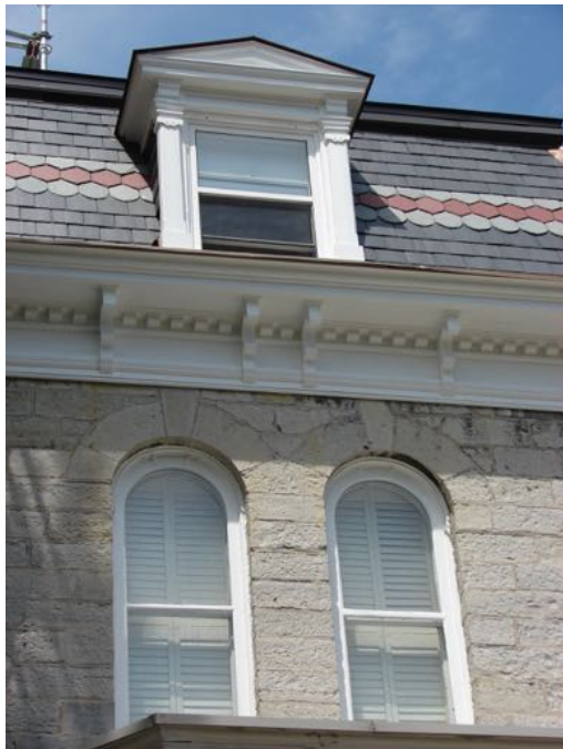
151 Earl Street—detail of windows, cornice, dormers and mansard roof/ Paul Christianson 2016
